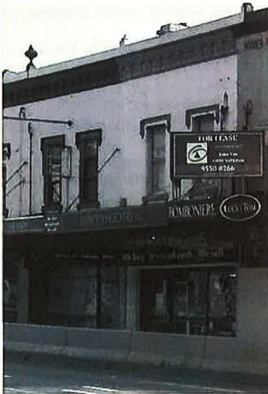
Figure 23 – Commercial building, c. 1880s; featuring painted surfaces and details in contrasting colours
