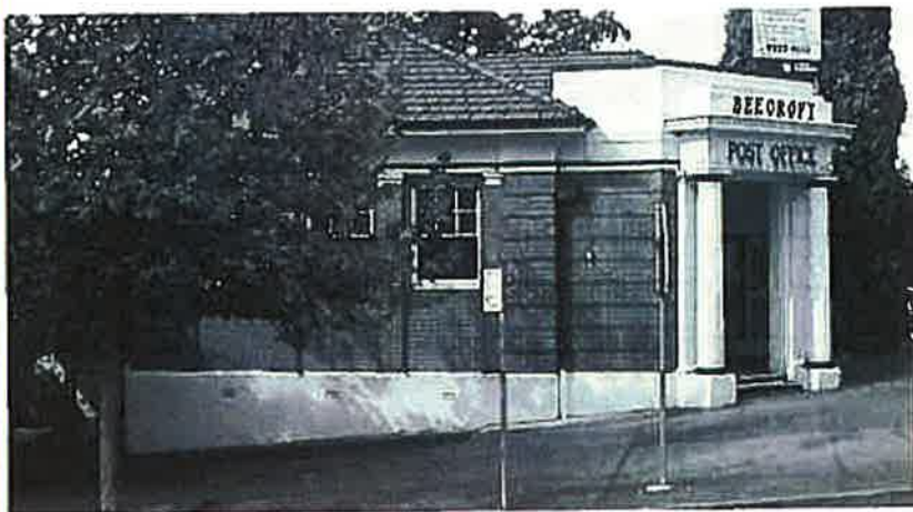
Figure 29 – Restrained interwar classical suburban post office building, c. 1930s; featuring carefully composed face brick with painted rendered decoration
