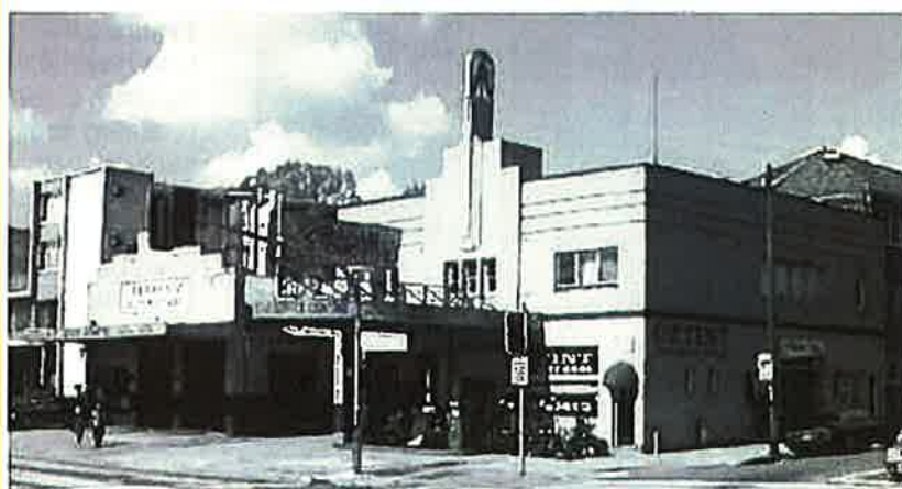
Figure 27 – Art deco garage, c. 1930s; featuring painted rendered walls and distinctive horizontal banded moulded decoration
