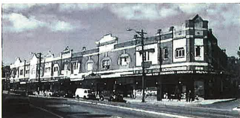
Figure 25 – Commercial building, c. 1910s; featuring some sections with painted face brick
